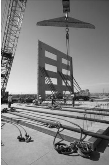
Figure 7. Tilt-up Wall
